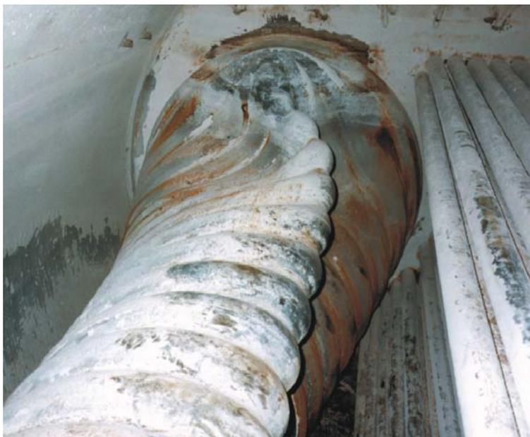
**Fig. 1** Thin silicate scale on a fire tube of a shell boiler led to a severe fire tube deformation due to over heating
